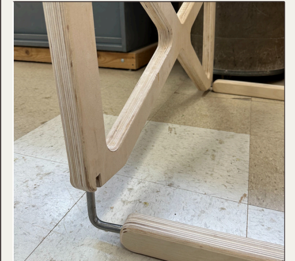
ensuring joint was flush and frame is properly balanced
